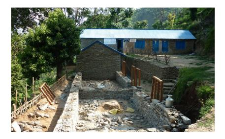
This photo was taken in late June 2010. It has been included to illustrate the construction methods used in Nepal. The walls are simple stacked stone sourced locally.
